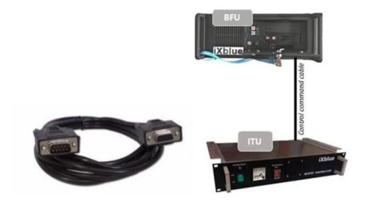
ITU↔BFU Control Command cable shall be terminated during the installation as per the following instructions.
